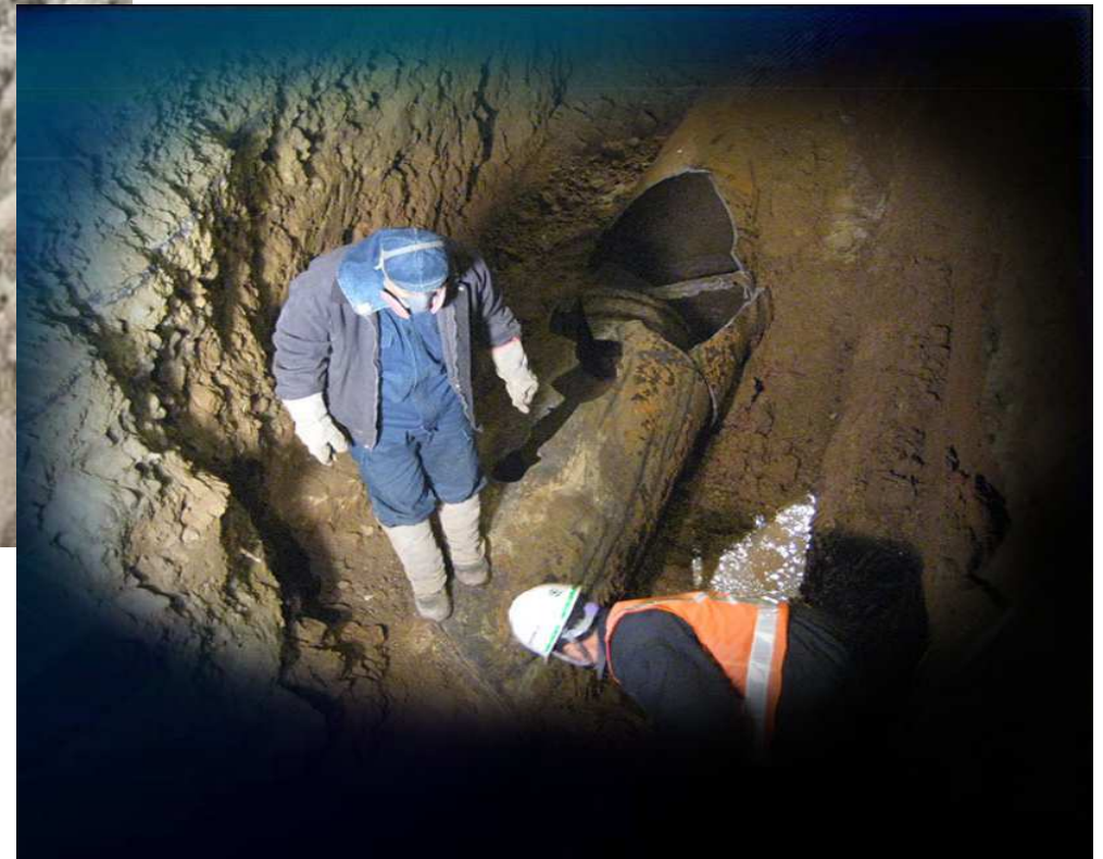
Existing underground utilities within depth of trench
