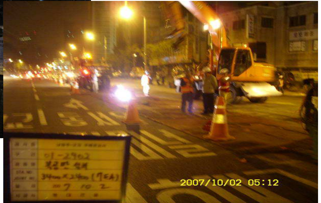
Road surface restoration at night
