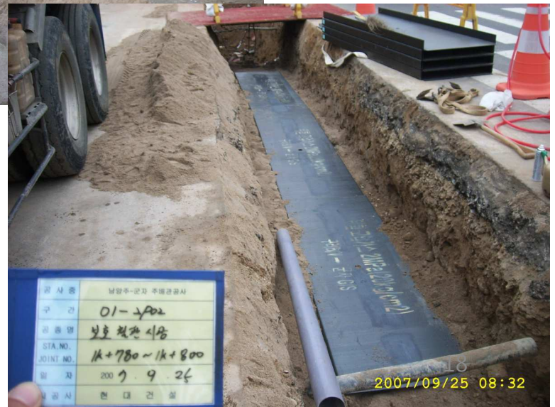
Steel plate installment
