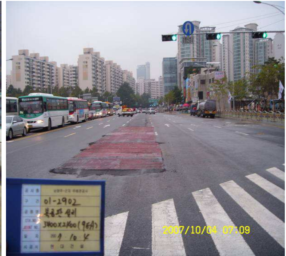
Covering with Steel plate on the road
