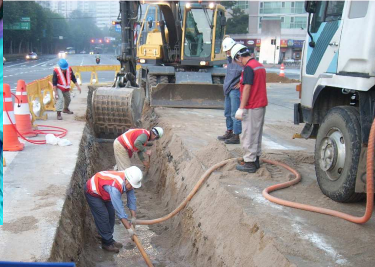
Compaction by watering (water binding)
