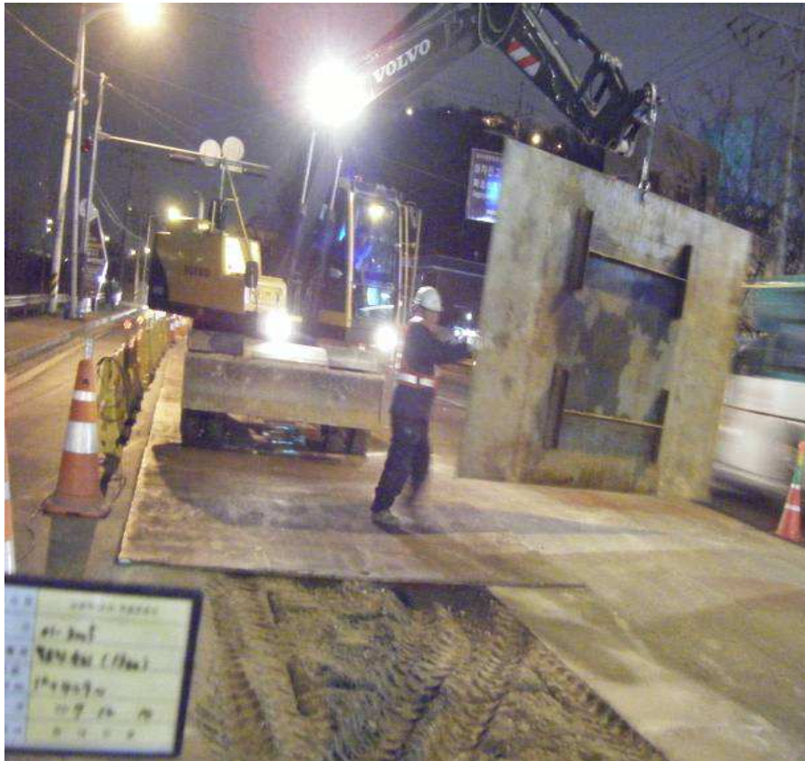
Backfilling in U/G welding Joint area
